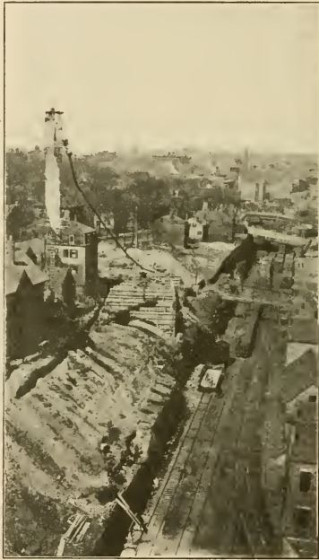
FIG. 3. CONSTRUCTING SECTION 6, TYNG STREET TOWER AT LEFT.
